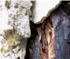
Non-friable asbestos may become friable after being exposed to fire
