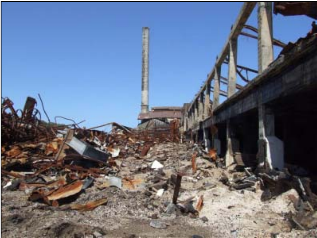
Photograph 1 Part of the site after the fire and prior to demolition
