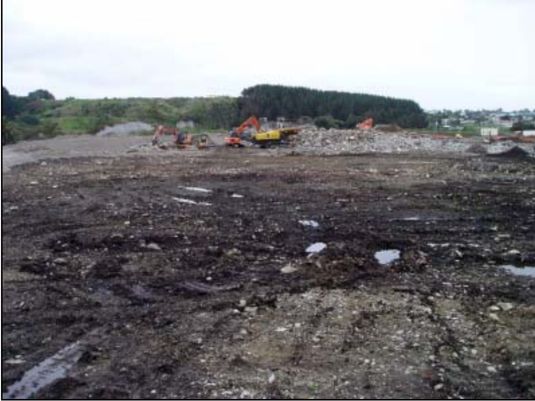
Photograph 2 View from east to west on 3 May 2010
